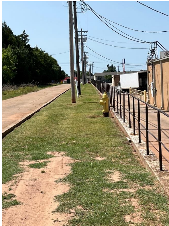
Fire Hydrant along the well line to Reno.
