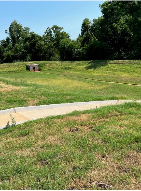
Detention Pond Improvements
