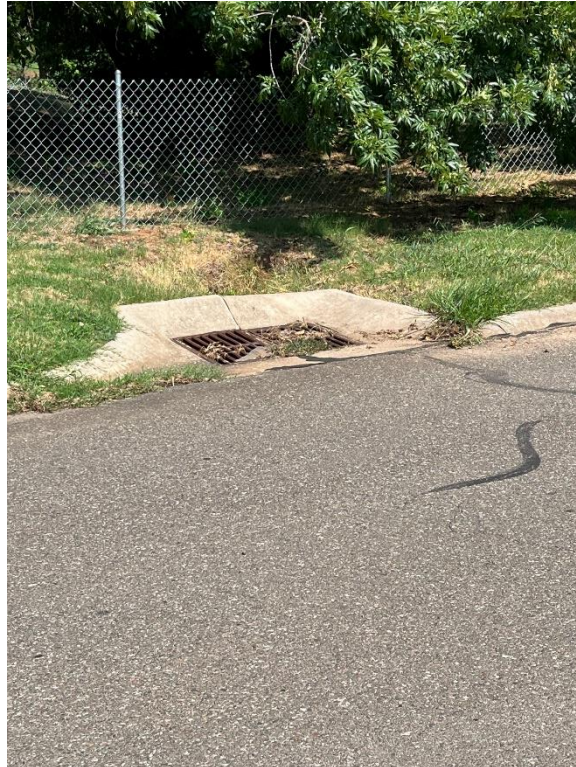
Drainage structure the detention will tie to.
