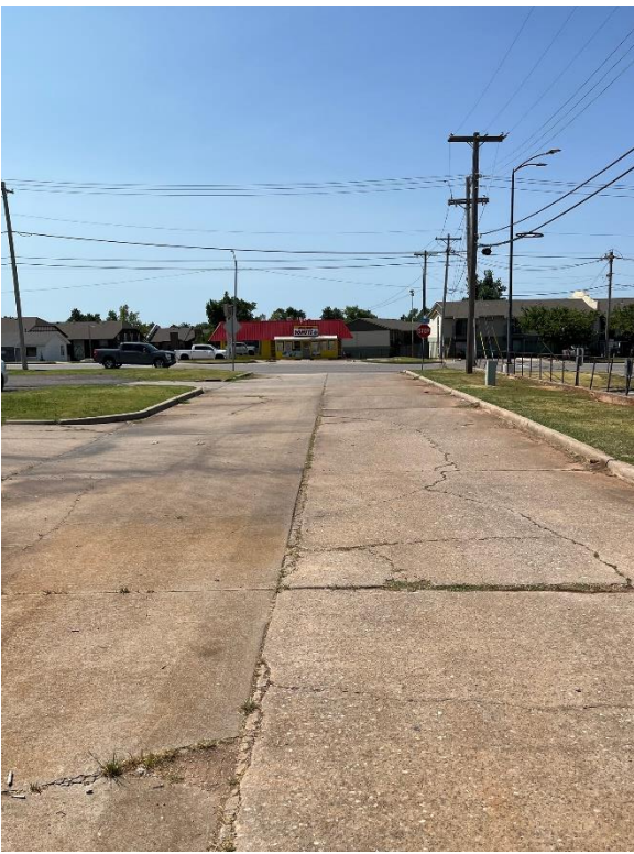
Marlow Drive – Reno Avenue intersection
