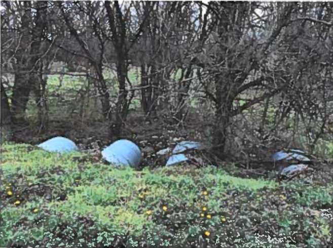
Outfall of west pond looking downstream
