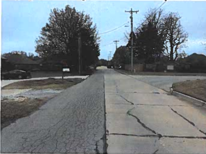
Looking south on Davidson Dr. Example of half street improvements on one side eventually being improved by another half street improvement further south.
