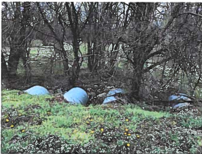
Outfall of west pond looking downstream
