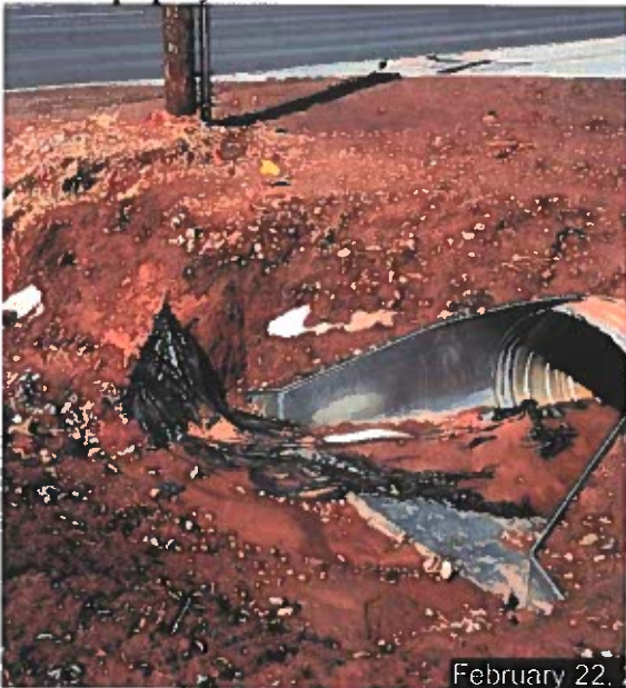
Upstream end of drainage culvert going under newly constructed driveway for Lot 1
