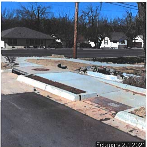
Sidewalk on northern end of property
