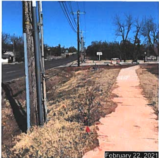
Looking north along N Douglas Boulevard from midway
