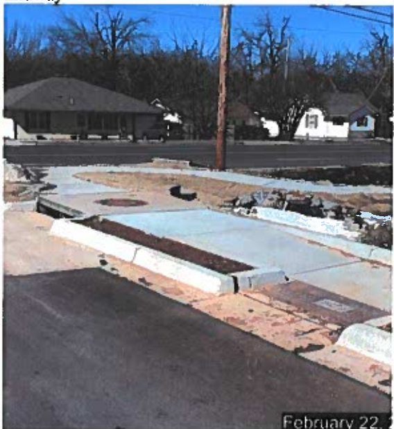
Sidewalk on northern end of property
