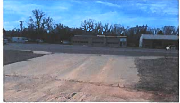
Existing drive on Douglas in the middle of the property, approximate location of StatusOne Dr.
