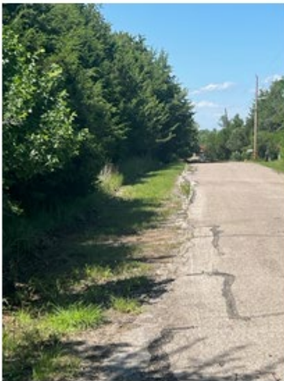
South along Randolph Ave
