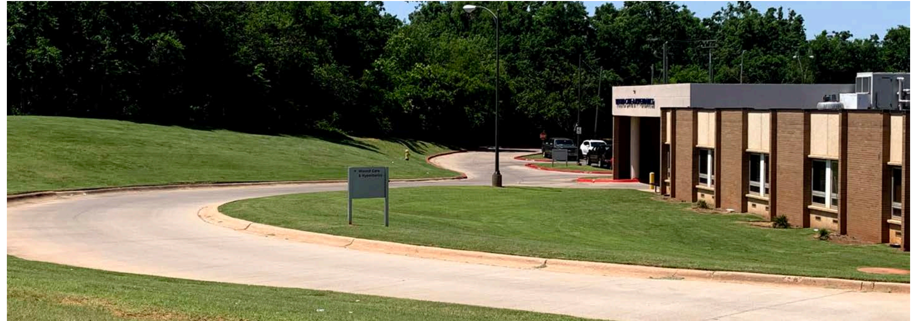
Top image: Existing topography that drains toward the channel behind the hospital along the western edge of the project site.
