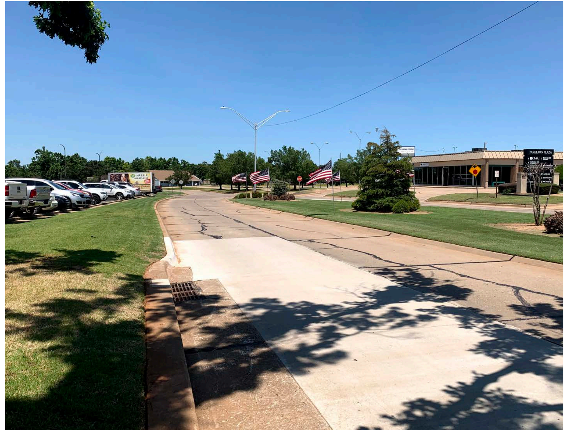
Looking north along Parklawn Drive
