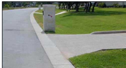
Illustration 3-28 RIBBON CURB (A Type of Sloping Curb)
