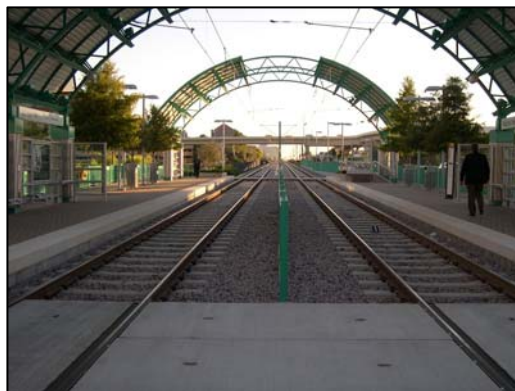
Illustration 3-22 EXAMPLE OF ADAPTING AN ABANDONED RAIL LINE TO SERVE AS A LIGHT RAIL LINE (Dallas, Texas Region)
