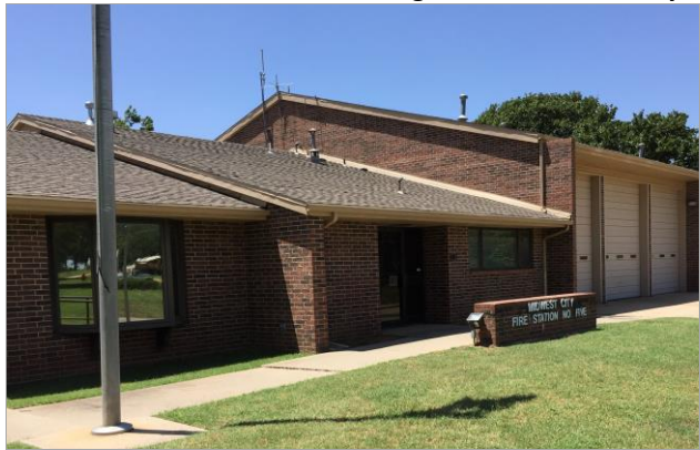
Figure 47: Midwest City Fire Department Station 5
