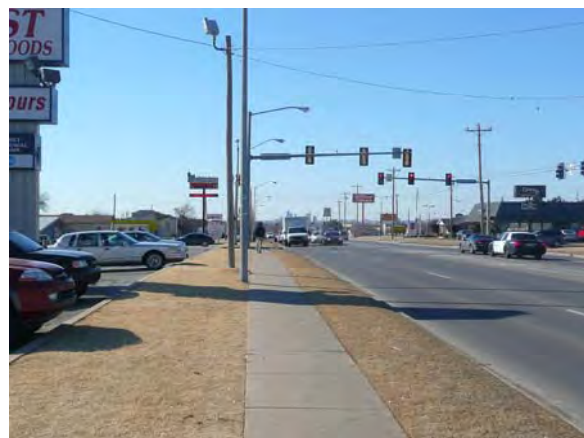
Exposed pedestrian conditions with no traffic buffers
