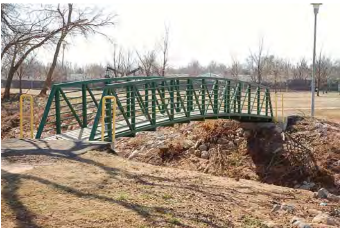
Safe and access able crossings
