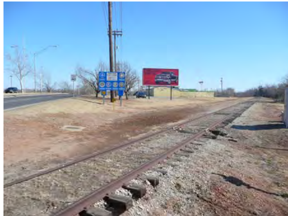
Rail Corridor at Reno
