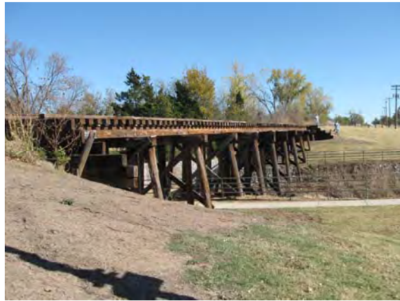
Rail Crossing and Underpass at Quinlan Park
