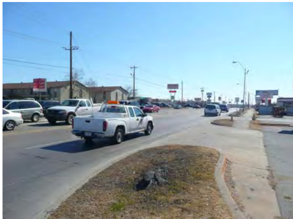
Pedestrian Obstructions, Driveways and Curbs
