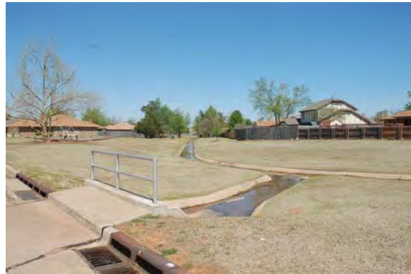
Wide ROW, Trib 6 off 15 th Street
