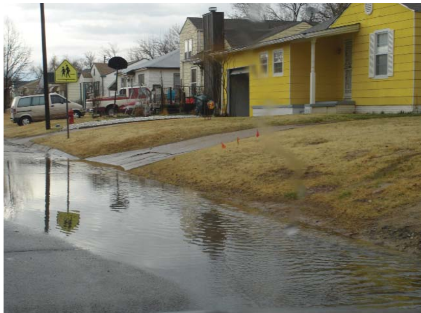
Flooding due to inadequate curb and gutter
