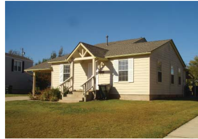
Example of sound housing condition
