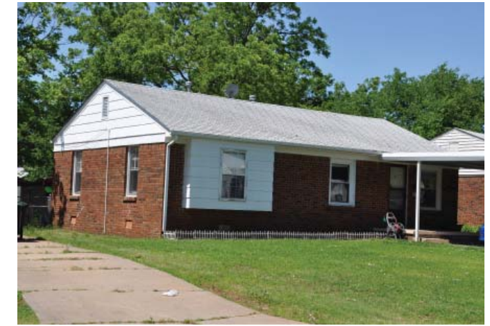
Example of sound housing condition
