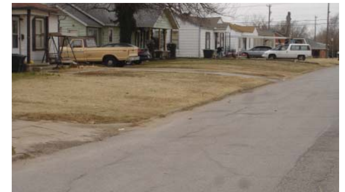
Asphalt overlay with “disappearing curb”
