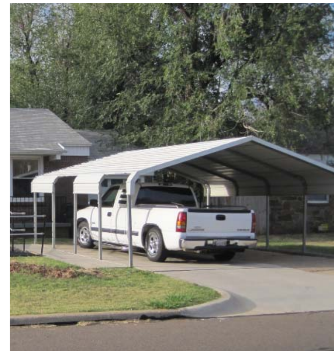
Example of existing metal carport
