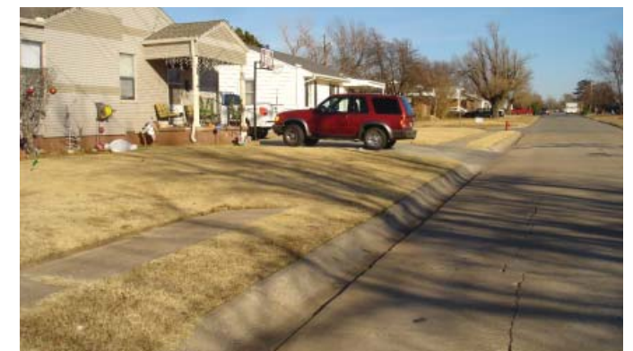
Original concrete street and mountable curb
