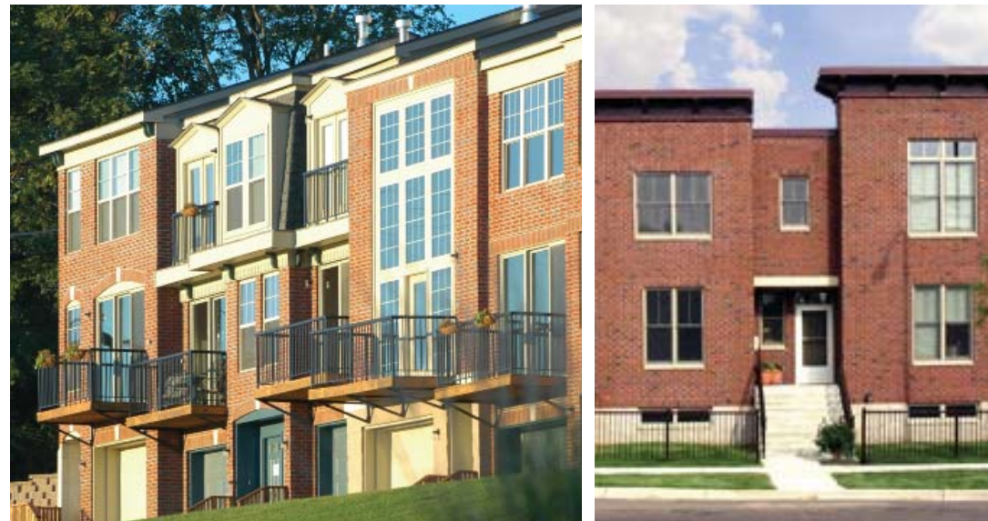
Examples of brick facade rowhomes
