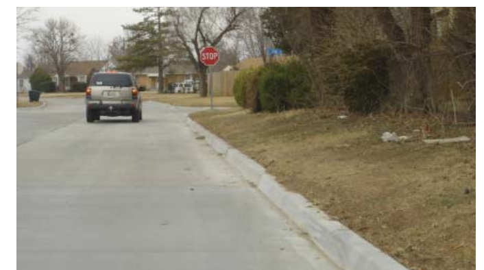
New concrete street and barrier curb
