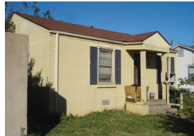
Example of deteriorating housing condition
