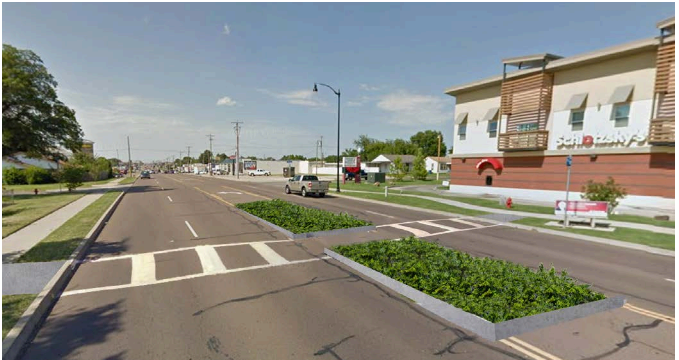
Below: The image below illustrates a mid-block crossing along Air Depot Boulevard, consisting of a pedestrian crosswalk and a landscaped median. These strategies can serve as a traffic calming technique and enhance safety for pedestrians.
