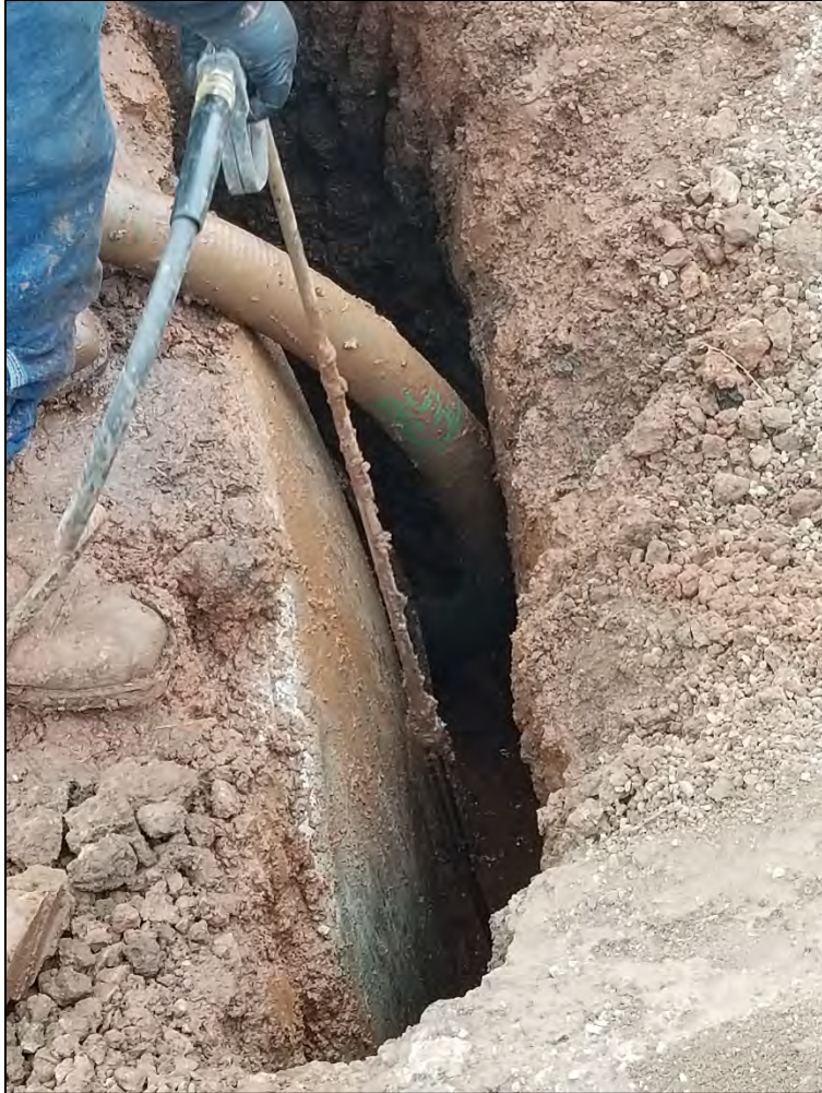
Potholing on West End of UST 12/18/17
