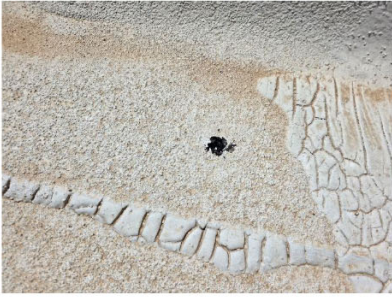
Photo #20 Roof tar
