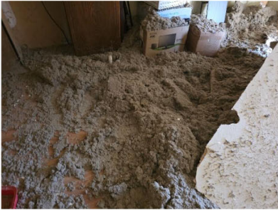
Photo #3 Ceiling insulation
