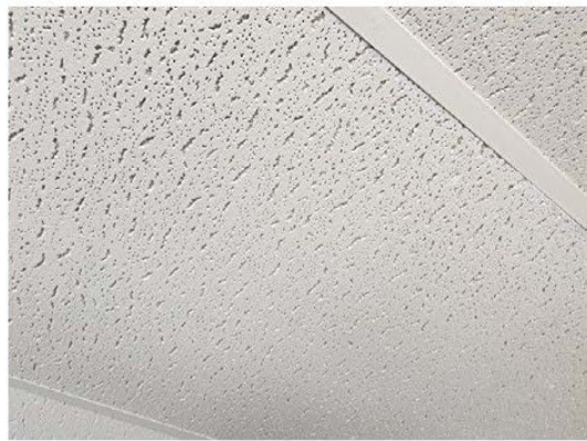
(I-03) No Asbestos Detected
