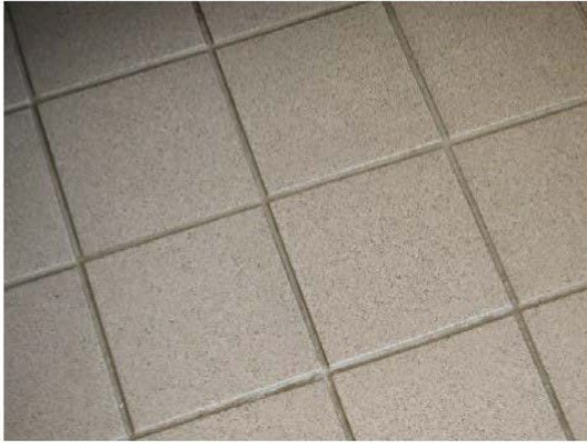
(H-08) No Asbestos Detected
