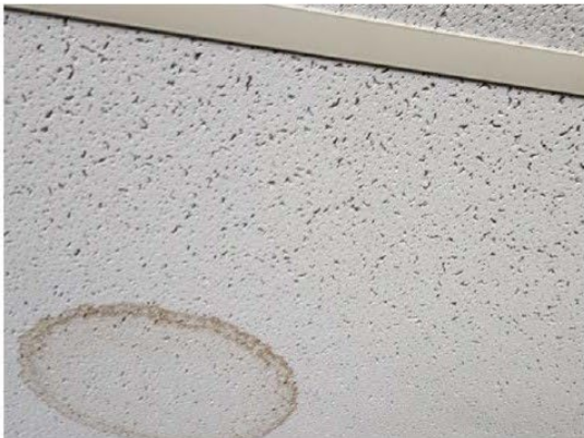
(I-04) No Asbestos Detected
