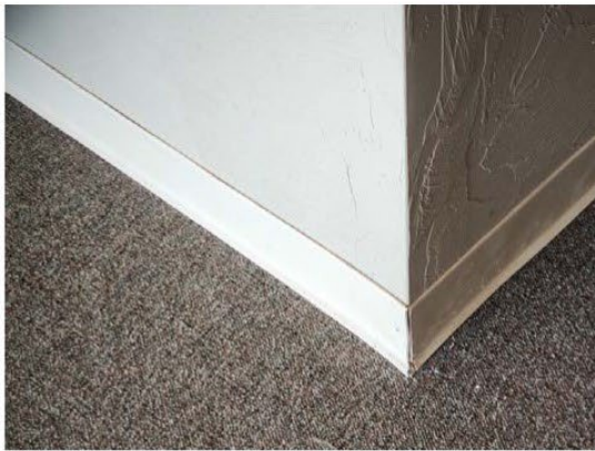
(I-06) No Asbestos Detected
