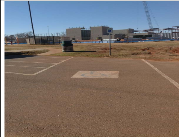
5. Comments: Violation AR_I2
