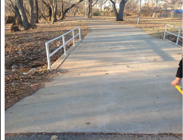
1. Comment: Violation AR_I1
