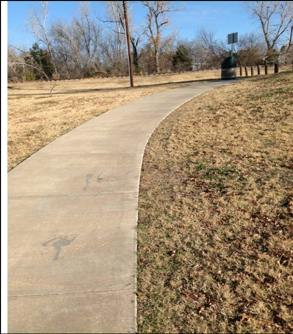
1. Comment: Violation AR_I1
