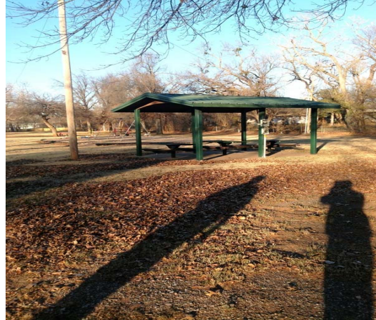
8. Comment: Violation Amn_11
