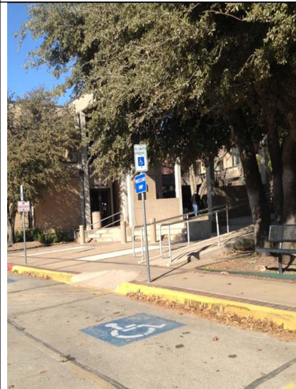
3. Ramp on south side of City Hall
