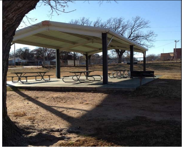
3. Comment: Violation AR_I1
