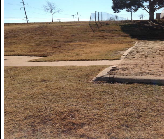
7. Comment: Violation AR_I5
