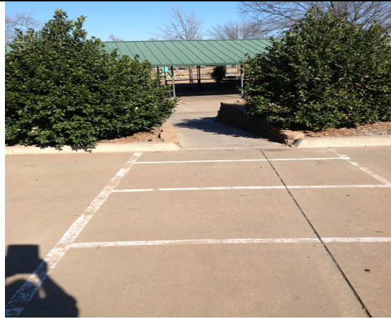
2. Comment: Violation AR_I2
