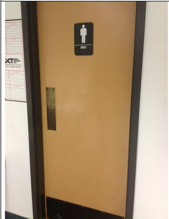
15. The signage is required to be mounted on the latch side of the door with both raised characters and Braille.
