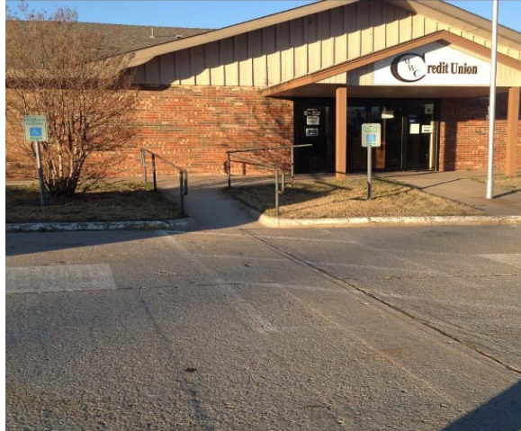
2. Comment: Violation PL_I2
