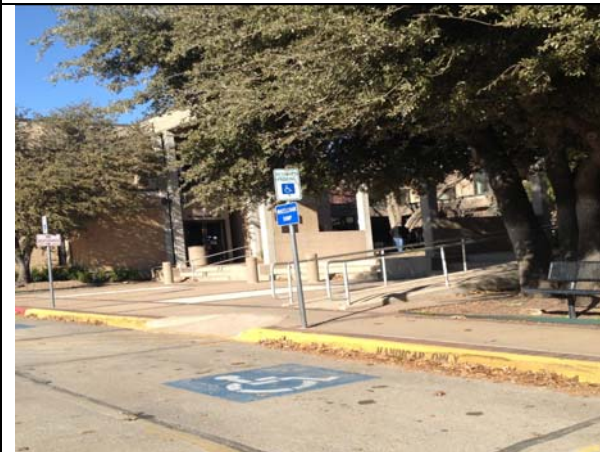
3. Comment: Violation PL_I3
