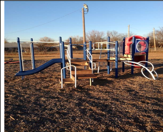
3. Comment: Violation MS_I1
