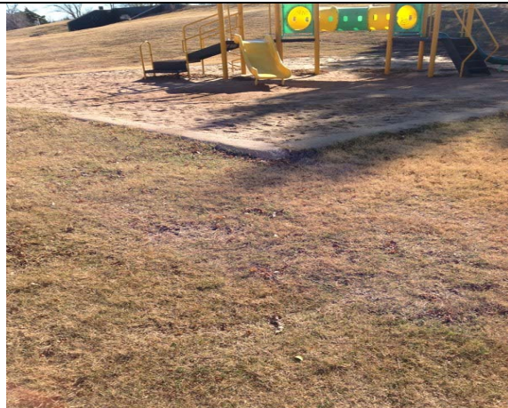
6. Comments: Violation AR_I3
