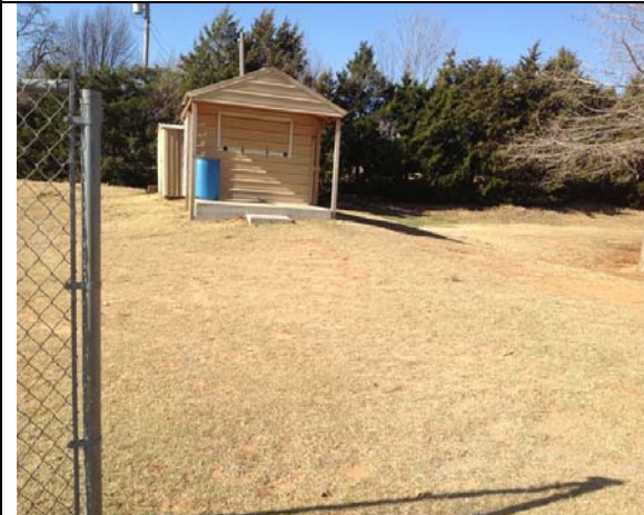
3. Comment: Violation AR_I1
