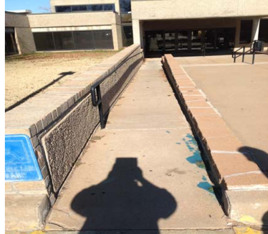
2. Entry ramp with one handrail.
