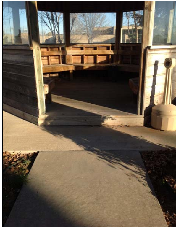
4. Employee gazebo north side of City Hall
