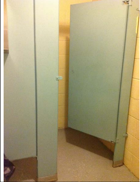
5. Women's restroom partitions can be removed
