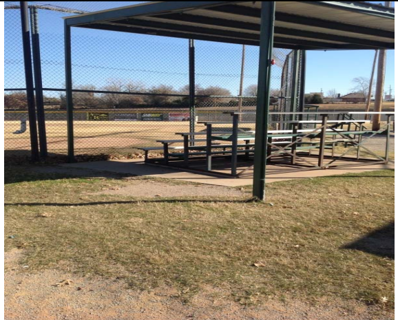
8. Comment: Violation AR_I6
