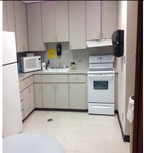
18. No Knee clearance under break room sink
