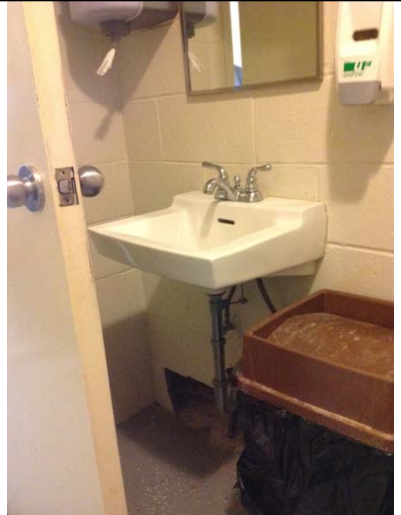
4. Men's restroom, door swings into clear floor space requirements
