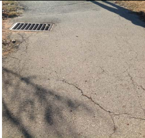
9. Exterior path of travel.
