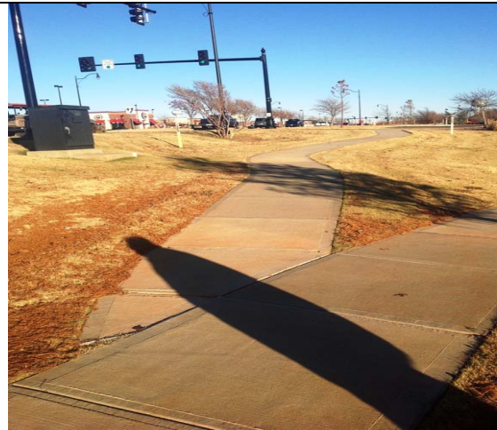
4. Comment: Violation AR_I3
