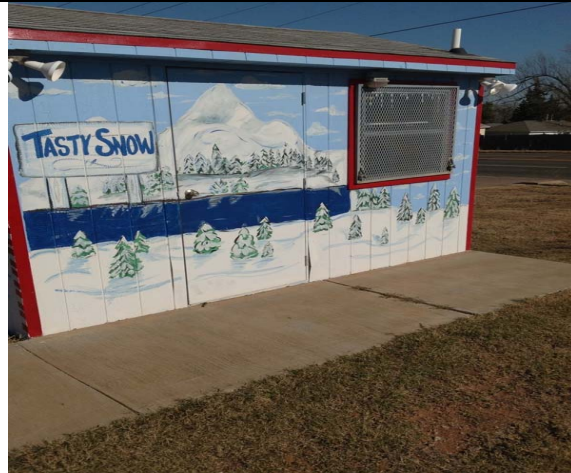
14. Comment: Violation Amn_I1
