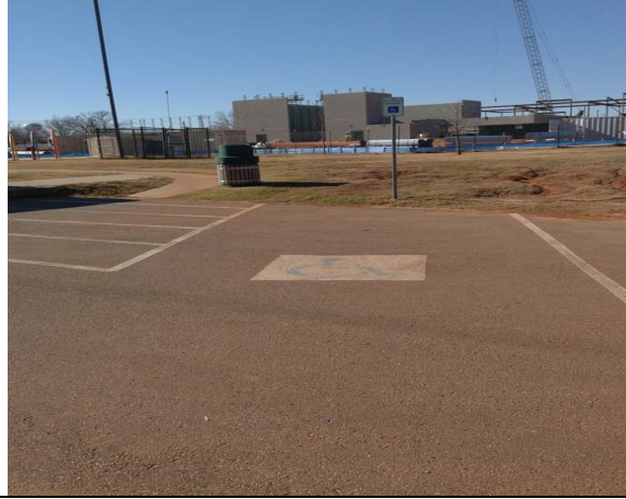
2. Comment: Violation PL_I2
