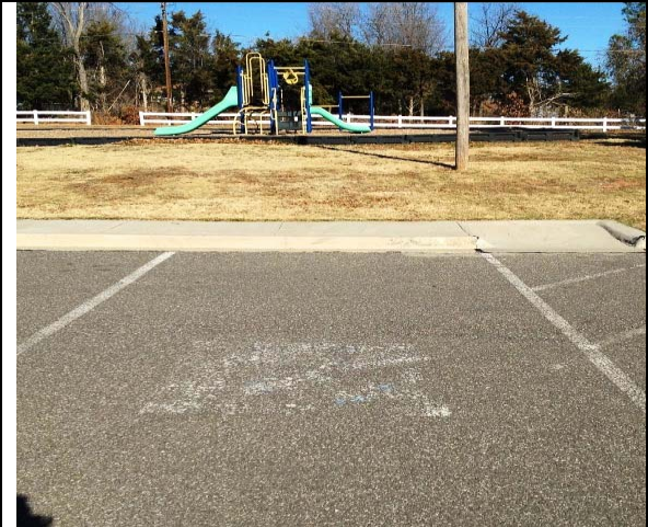
1. Comment: Violation PL_I1
