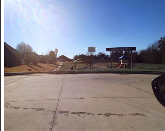
1. Comment: Violation AR_I1
