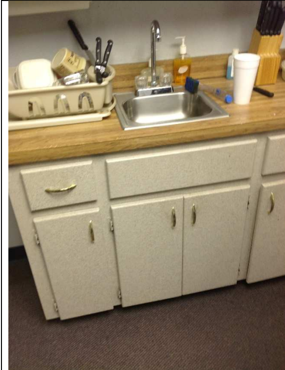
5. This break room is required to have counters at 34" and knee clearance under the sink.
