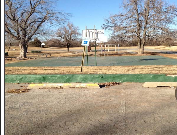
1. Comment: Violation PL_I1
