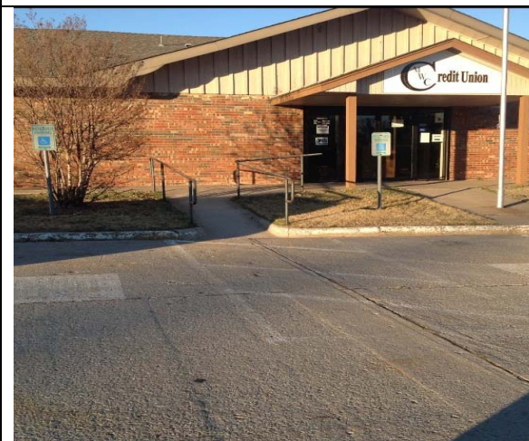
5. Comments: Violation AR_I3
