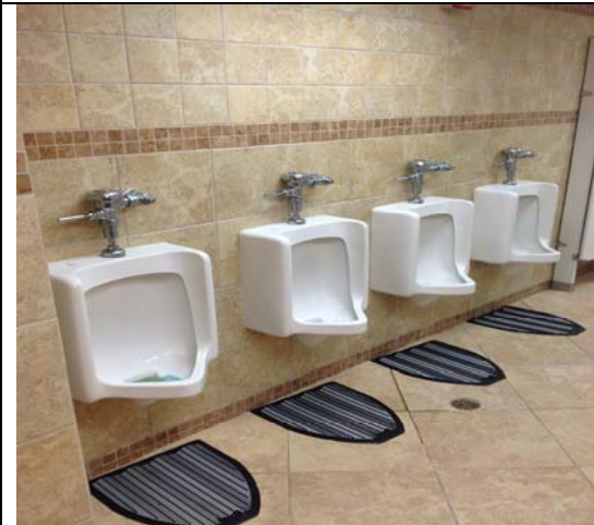
9. Men's restroom urinals.
