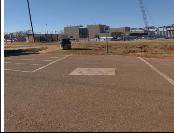
1. Comment: Violation PL_I1
