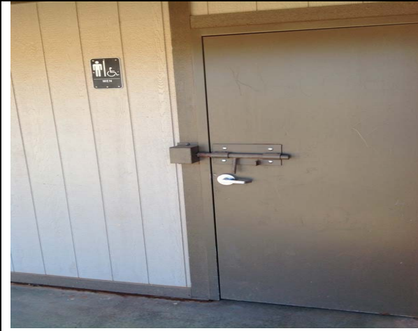
13. Comment: Violation RR_I5
