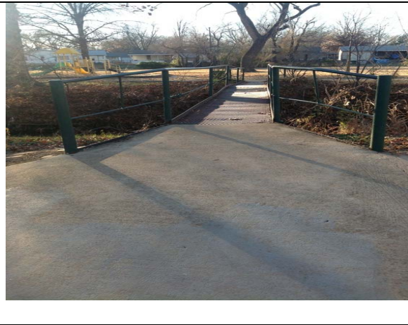
4. Comment: Violation AR_I4
