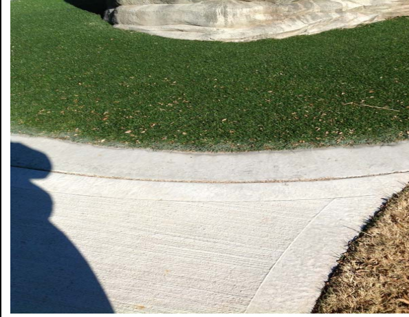
1. Comment: Violation Amn_I1
