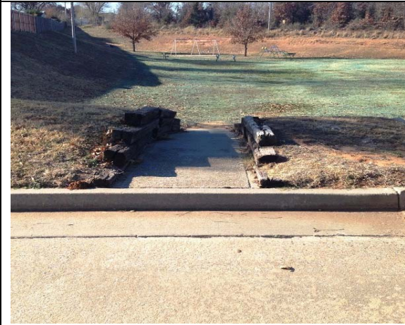
3. Comment: Violation Amn_I1
